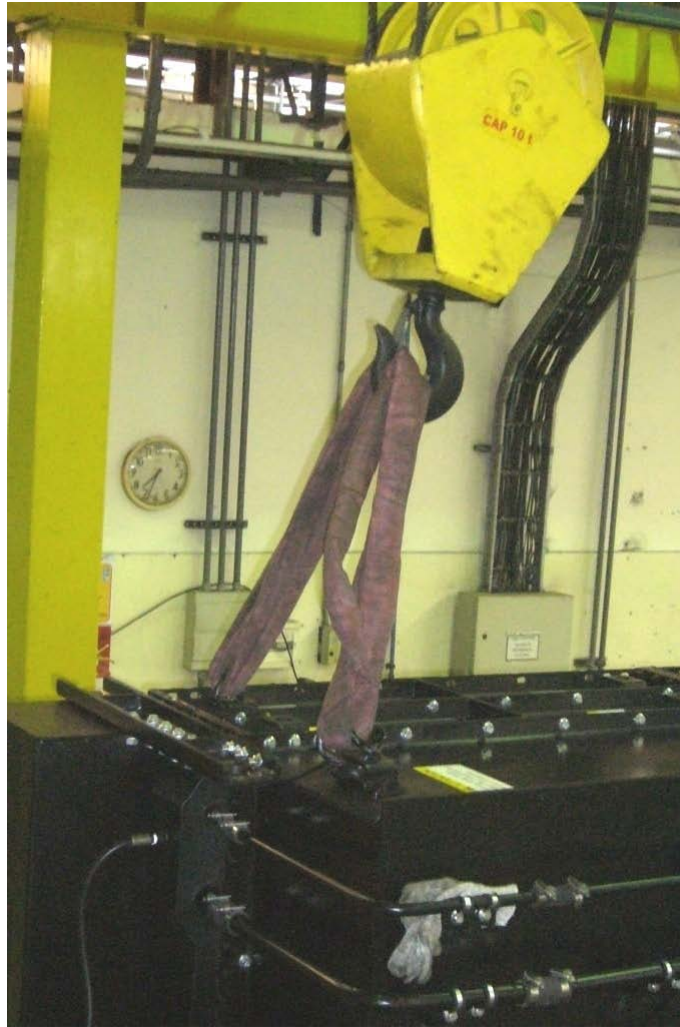
FIGURE 39. RADIATOR PREPARED FOR LIFTING
